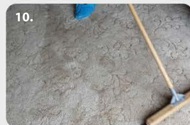
10. Set pile - Lay fibres flat to speed drying.
